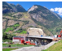
A9 motorway – Raron (CH)
