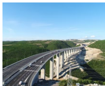
Liman Viaduct (TR)
