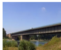
Rhine Bridge Frankenthal (DE)
