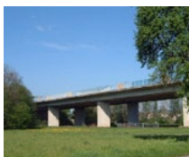
Ohrntal Bridge Öhringen (DE)
