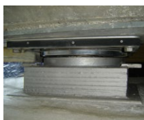
Spherical bearings
