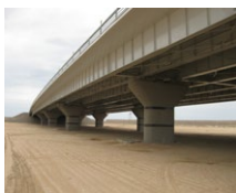
Awaza Bridge (TM)
