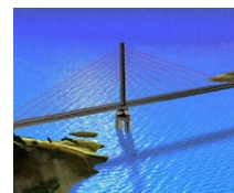
Agin Bridge (TR)
